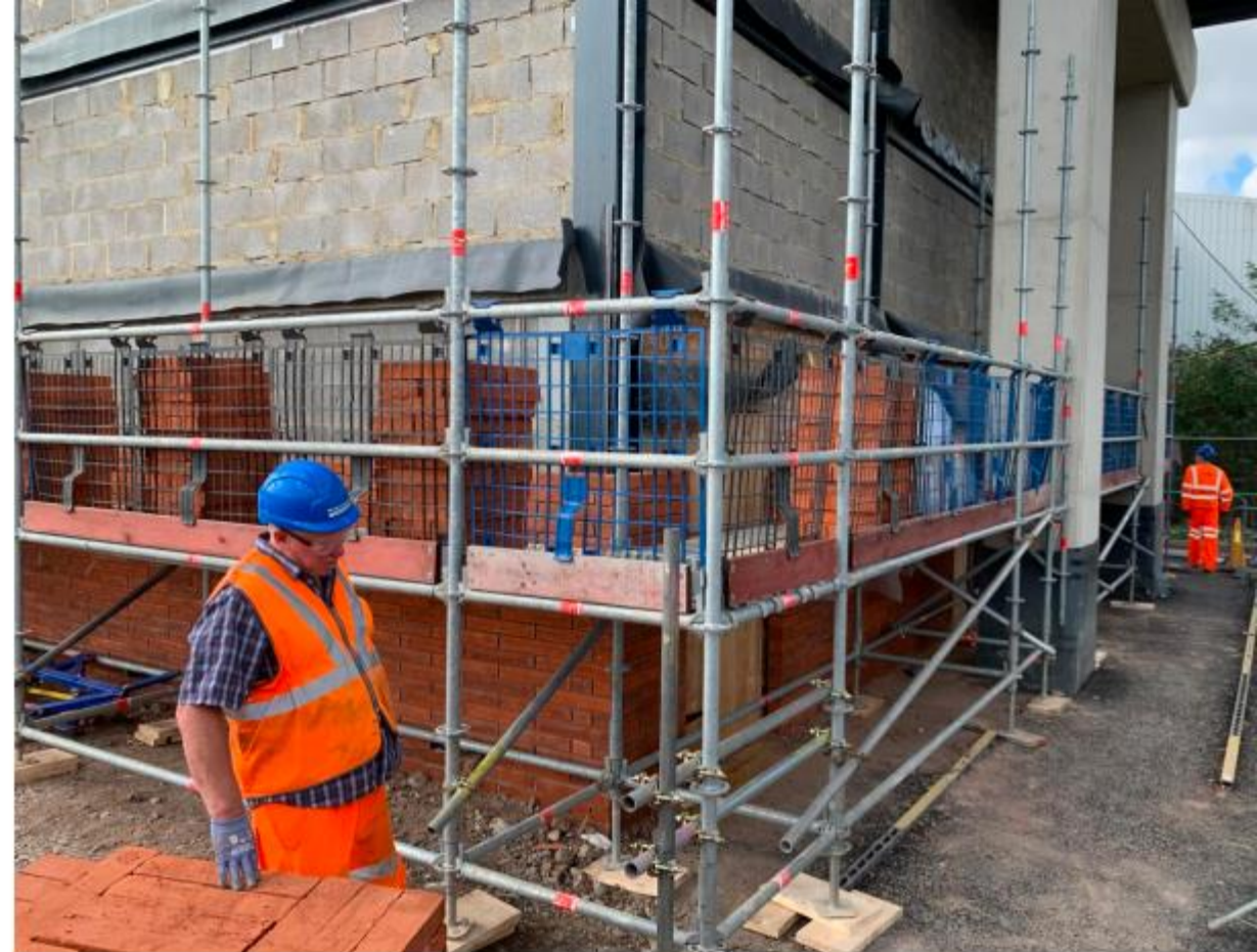
WEB brickwork onto the second lift
