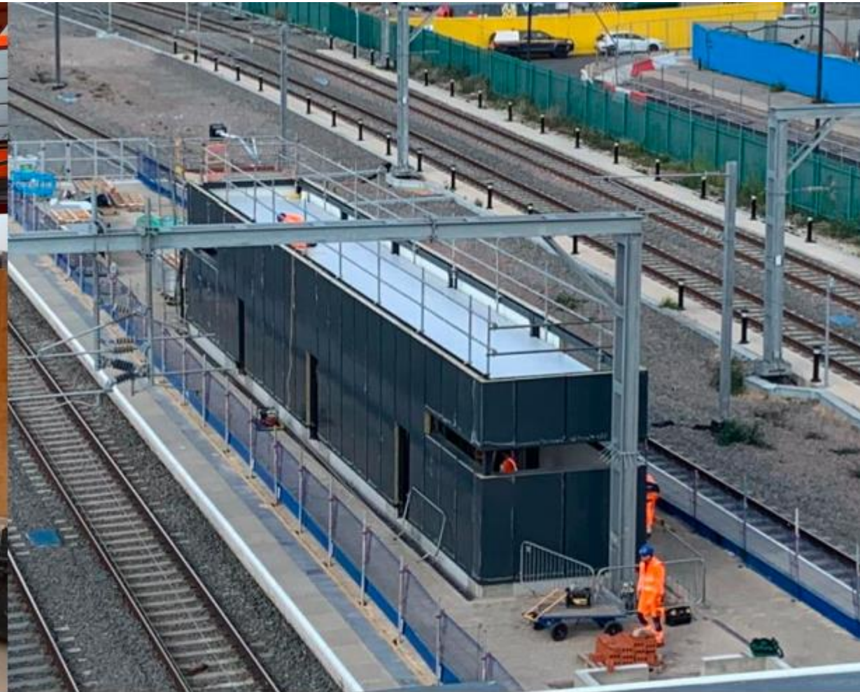
Drivers accommodation roofing installed
