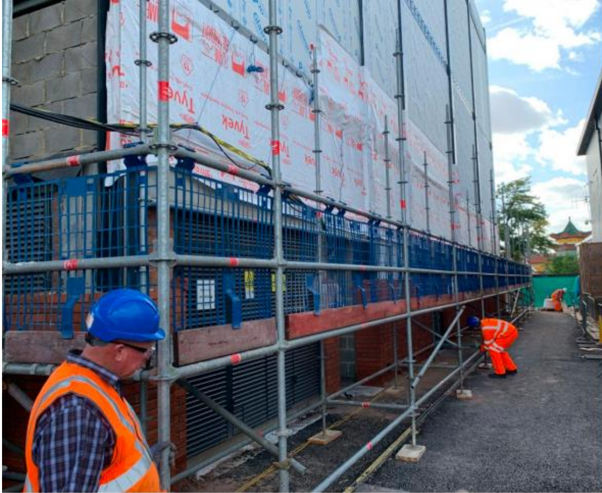
WEB brickwork onto the second lift
