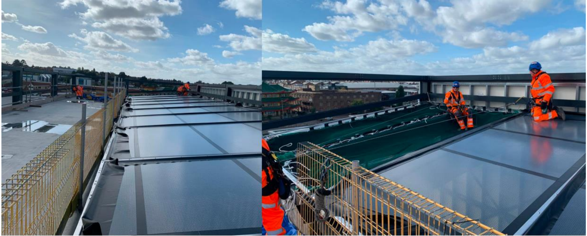
STFE roofing to the WEB
