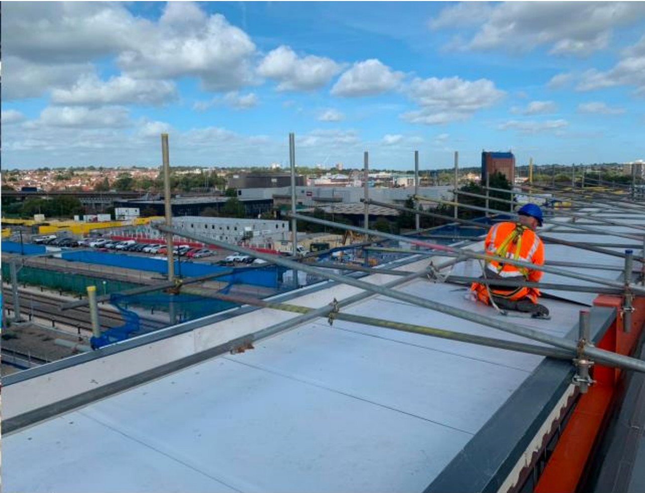
GL:1 roofing completed
