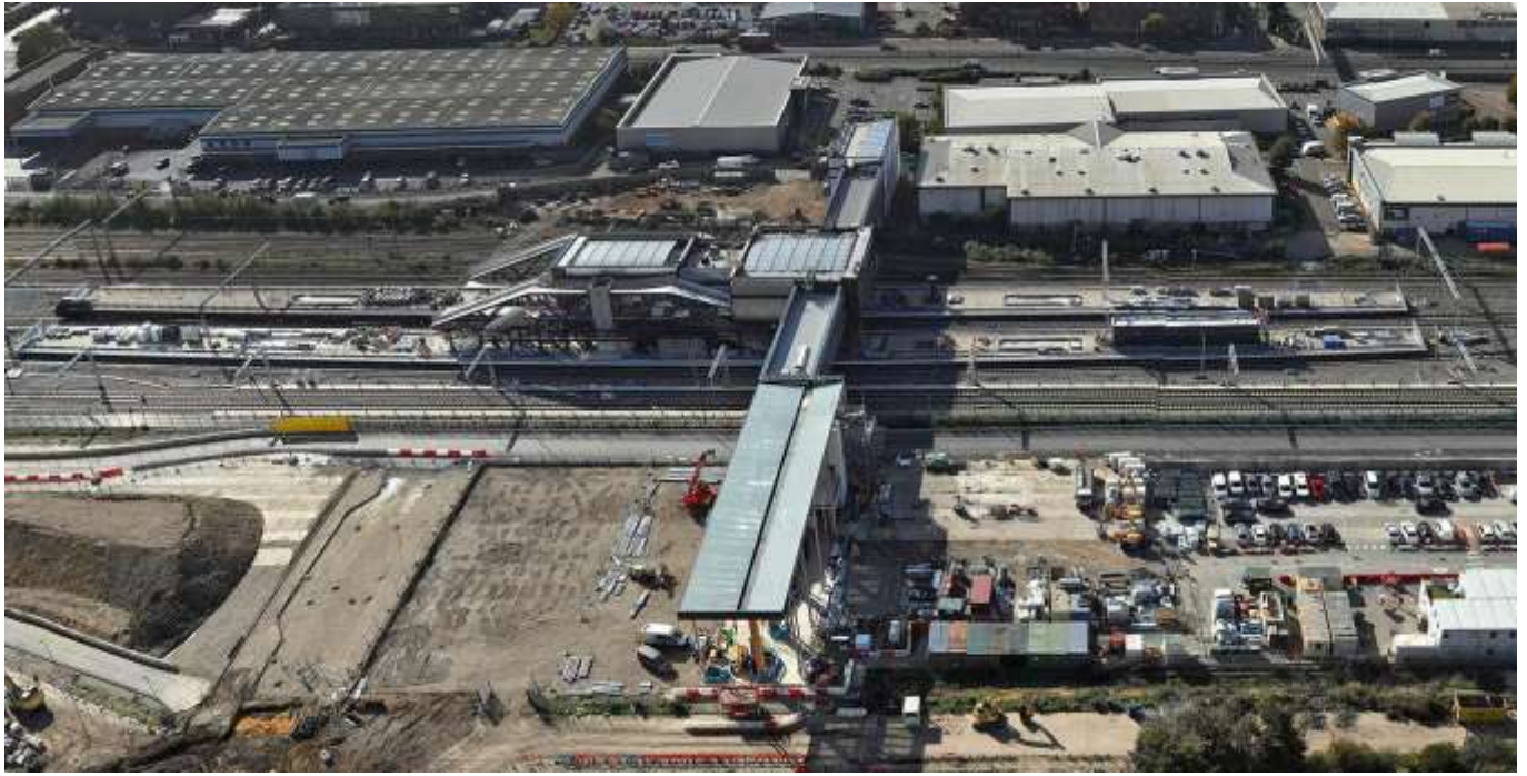
Figure 1 - Brent Cross West Station (October 2022)
