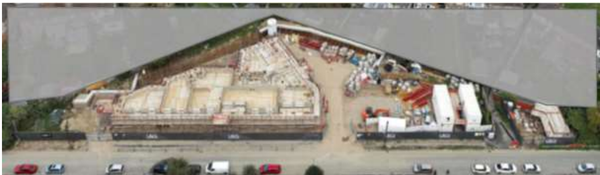
Plot 54 construction – October 22
