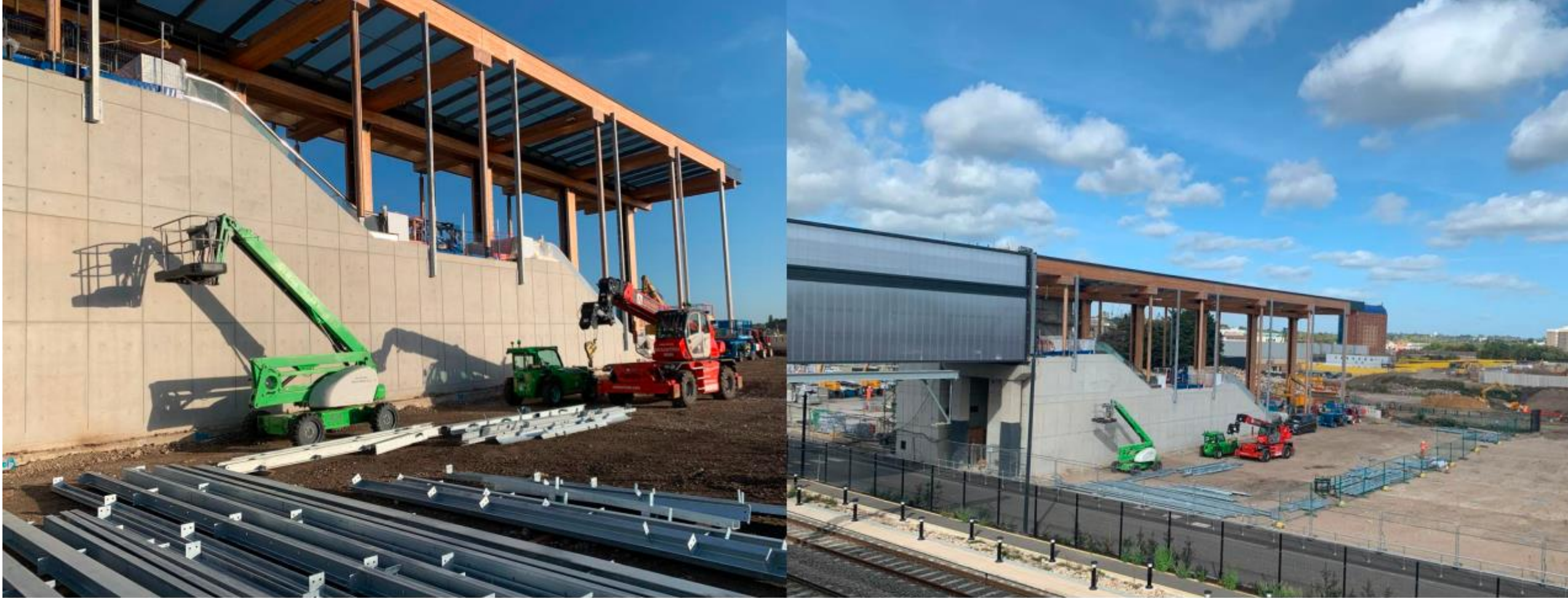
SEEB south elevation hoarding materials laid out ready to commence
